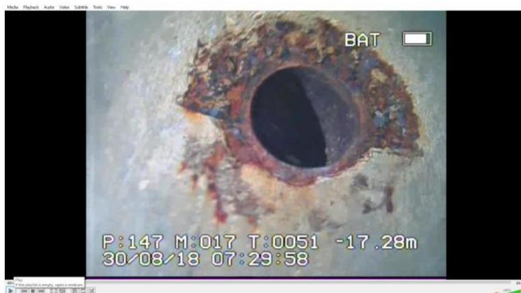
**Problem:** As part of a program to upgrade the testing tank facility it was necessary to replace the valves on the southern end of the tank, these valves had served for decades and may now not function as a reliable method of containing the water in the tank.
